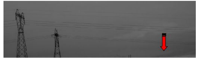
Fig. 7 Creep behavior of overhead aerial power line conductors.
