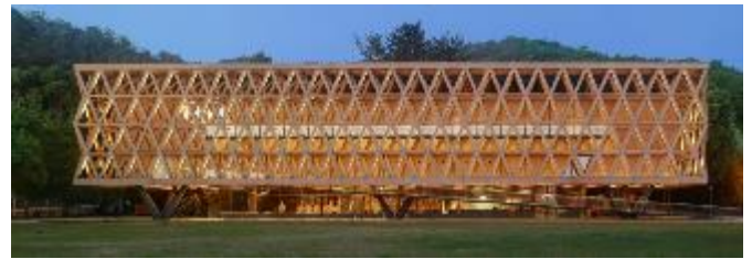
Fig. 5 Chile Pavilion by by Undurraga Devés Arquitectos [6].
