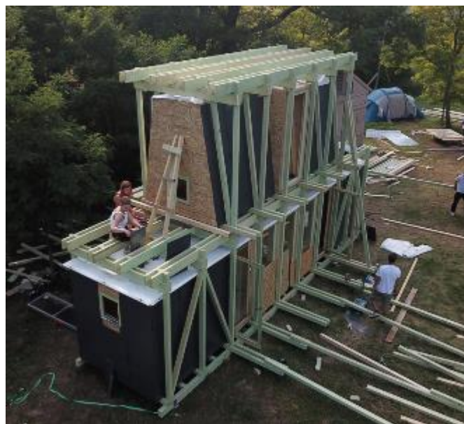
Fig. 28 Towards the completion of the construction of Ziggurat.
