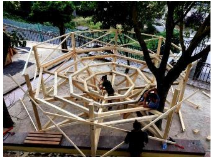
Fig. 13 The beams and braces for fences fitted on the structure.
