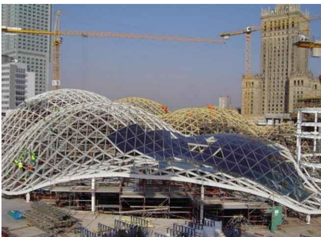
Fig. 3. Jerde Partnership International, The Golden Terraces, Warsaw, 2000-2007 – support structure under construction
