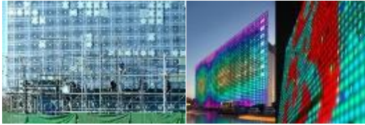
Şekil 11. Zero Energy Media Wall, Simone Giostra & Partners and ARUP, China, 2008.
