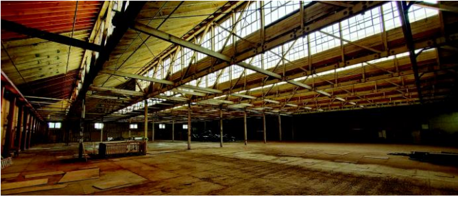
Fig. 1 The former Villa Park Orchards packing house [6]
