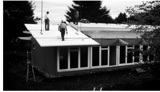
Fig. 5th Use of Blockholz panels on the roof of Wiki House [8]
