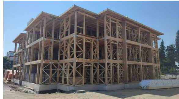
Fig. 14th Mass timber construction in the earthquake zone
