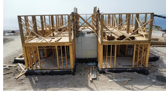
Fig. 13th Mass timber construction in the earthquake zone [25]
