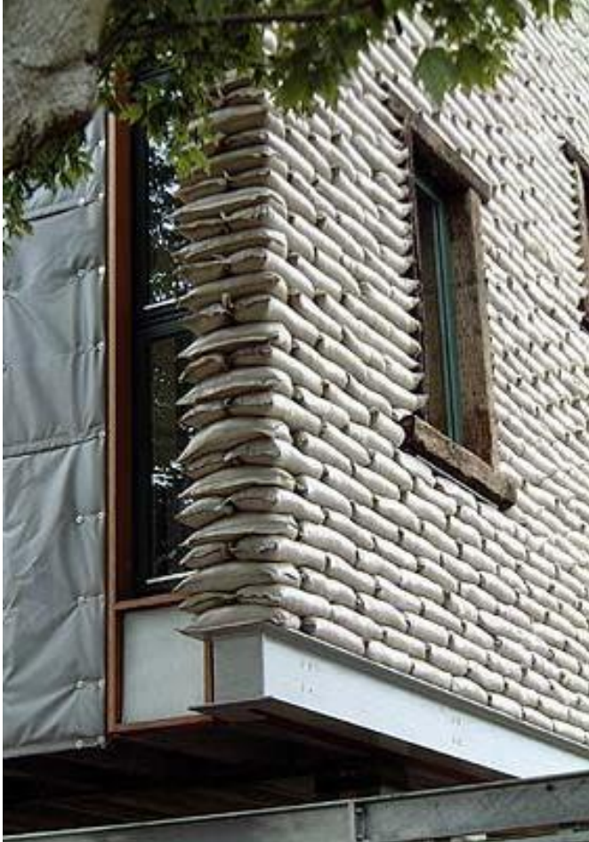
Fig. 16 Sarah Wigglesworth and Jeremy Till, Strawbale House , Islington, North London (finished in 2001). Detail of the facade facing the railroad, covered in bags filled with cement to mitigate the impact of noise.
