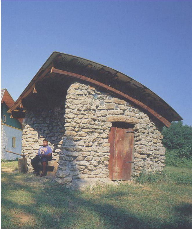
Fig. 7 Rural Studio, Bryant House, Mason's Bend, Alabama (2000). View of the storeroom with the cover obtained employing road signs discarded by the local Department of Transportation.
