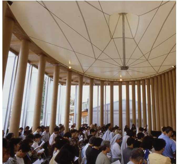
Fig. 11 Shigeru Ban, Community Center named Paper Church , Kobe (1995). View of the interior space and the cardboard tube structure recalling the shape of columns.
