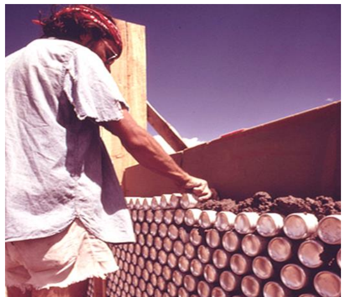
Fig. 4 Michael Reynolds, Beer Can House, Taos, New Mexico (1970s). Construction of a wall composed of a layer of aluminium cans.
