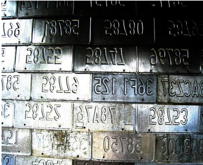
Fig. 9 Rural Studio, student housing at Auburn University's School of Architecture, Newbern, Alabama (1997-2001). Detail of the coating of the common restrooms made of old license plates.
