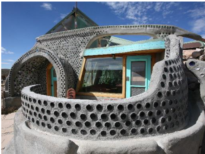
Fig. 5 Michael Reynolds, Phoenix House, Taos, New Mexico (2006). General view. The curved walls are decorated by the bottoms left exposed from the bottles and cans.
