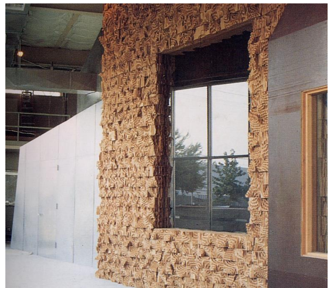
Fig.3 Frank O. Gehry, temporary offices of Chiat/Day, Venice, California (1986-88). Interior walls covered with blocks of cardboard.
